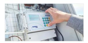
Manual: any action that is required immediately. For example, activate or stop a program, deactivate an alarm, make an emergency stop, etc.
